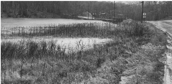
12/23/2022 South of Mill Creek looking towards Culvert prior to high tide incoming
