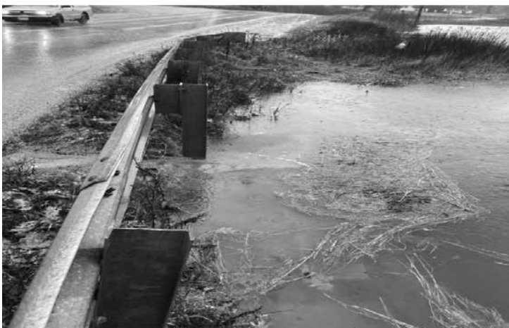
12/23/2022 Mill Creek culvert, downstream, prior to high tide incoming
