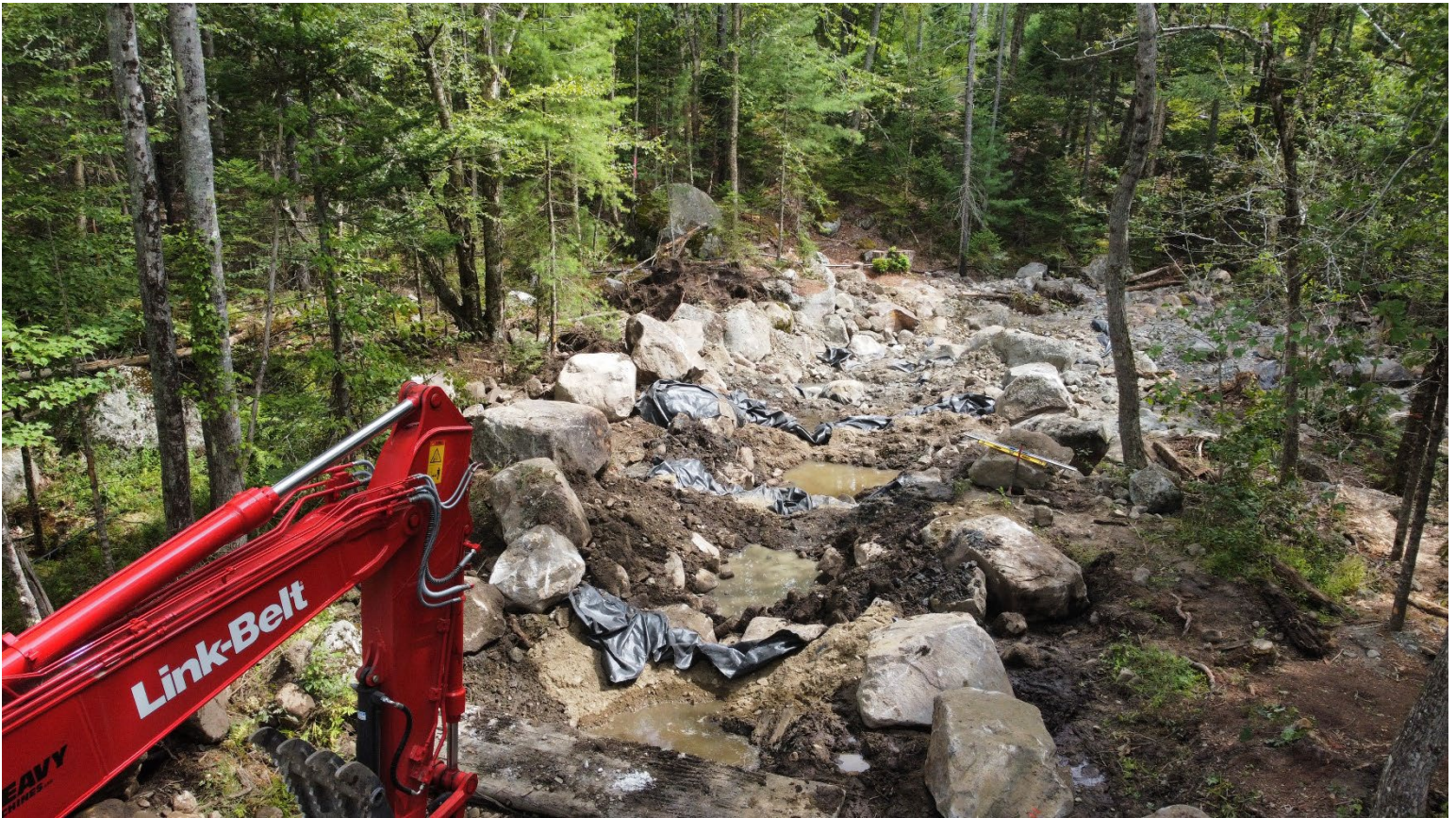
Photo taken 8/20 of most of the upstream portion of the work.
