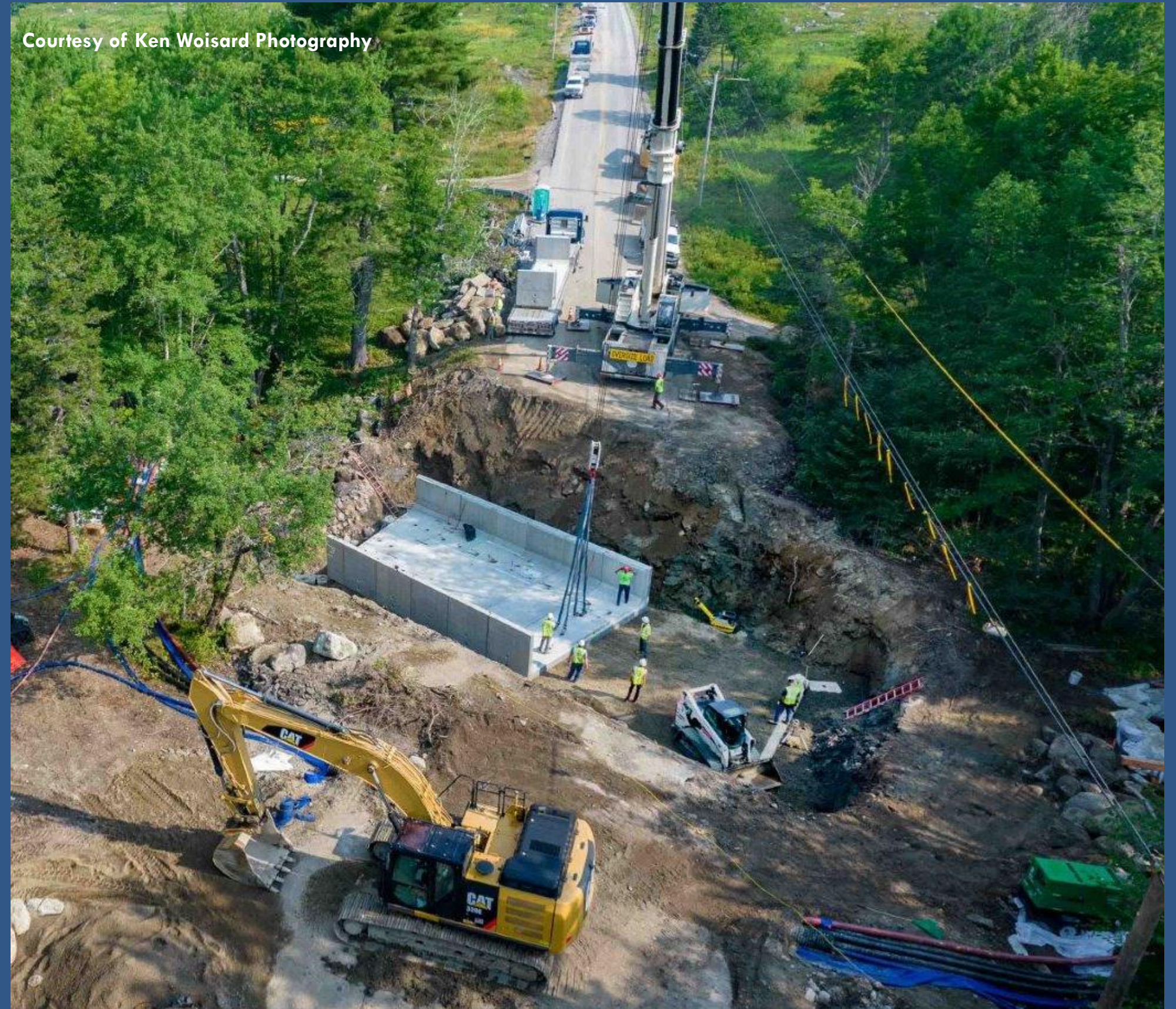
Snow Brook Culvert- Sedgwick, ME
